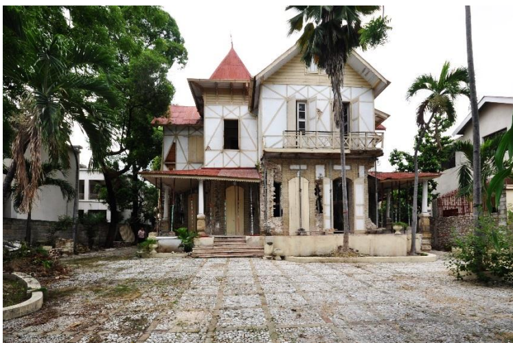
Figure 4. Maison Dufort in Port-au-Prince following the 2010 earthquake in Haiti
