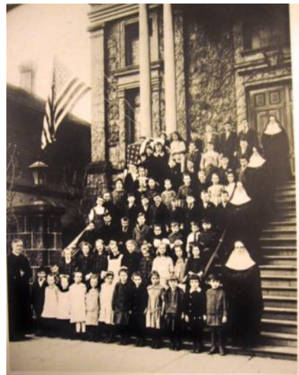
Original stairs St. Patrick's Church 1920. Image: St. Patrick's Church.
