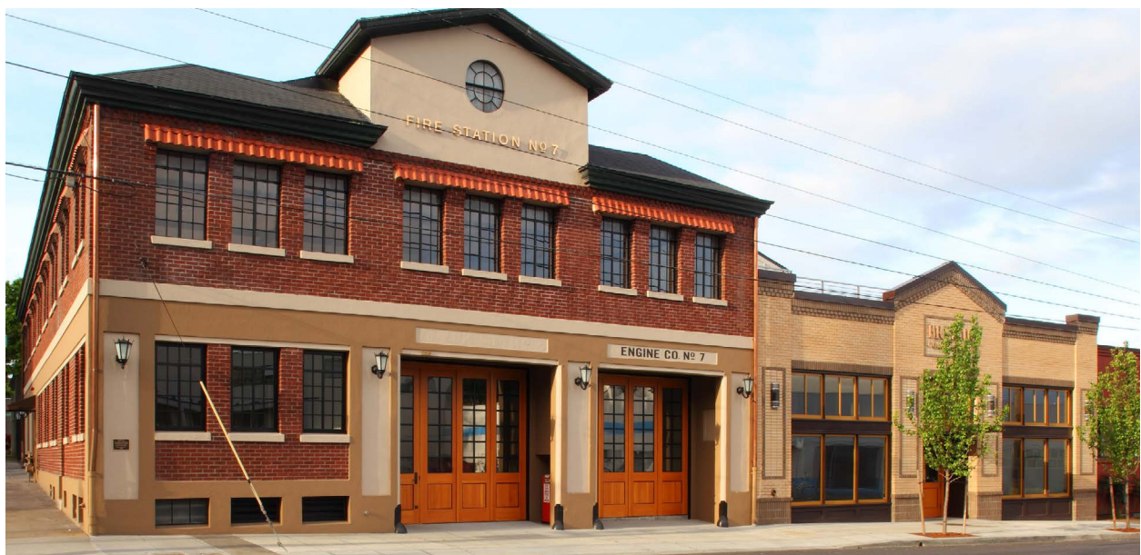
Federal Tax Credits were utilized for this conversion of an old Portland fire station into office space
