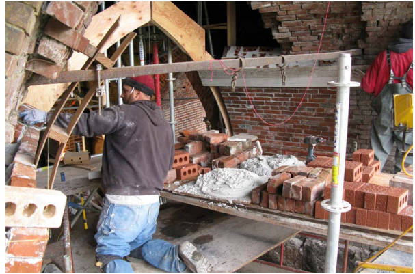
Oswego IronWorks arch reconstruction, Lake Oswego
