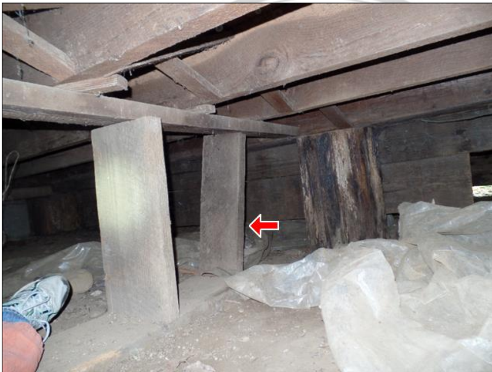
4.2 Item 2(Picture) Shifting support structure
