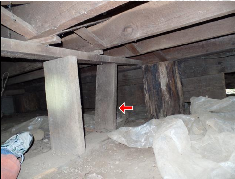
4.2 Item 2(Picture) Shifting support structure
