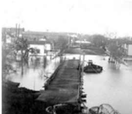
Photograph of the damage to the timber wagon bridge, looking north from Fry Hill in Salem, 1890. Photo courtesy of the Marion Co. Historical Society.
